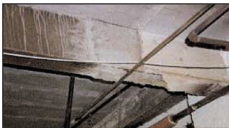
Steelwork coated with asbestos spray for fire protection.
