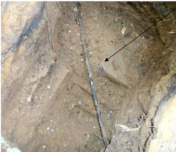
The photograph to the left shows the extent of the damage, and shows the lack of warning markings around the cable. There were no classic warnings around the cable for example, a layer of sand or yellow warning tape. The cable itself is leaded sheathed which provides no mechanical protection, so the slightest knock would cause a break.
