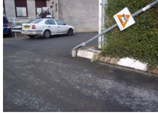
Damaged Lighting Column
