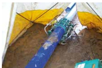
Butt welding working conditions
